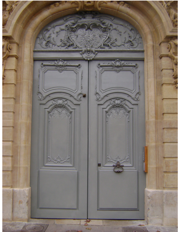
Restoration of 18 th century doors using linseed paint. Hôtel des Gendarmes, VERSAILLES.
