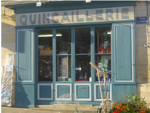
Restoration of 19 th century shopfront using linseed paint. Quincaillerie Mallet, Mirambeau, FRANCE.
