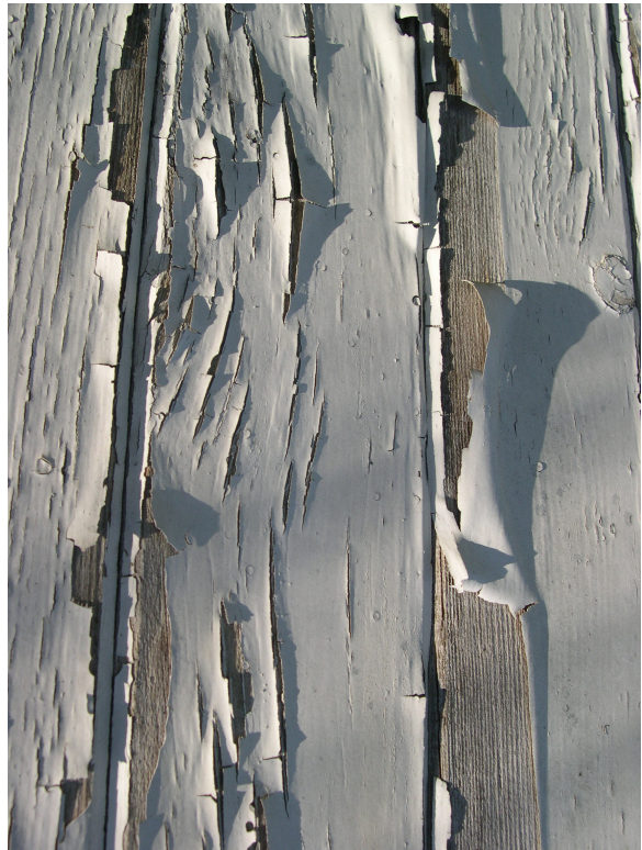
Typical example of modern paint failure.
