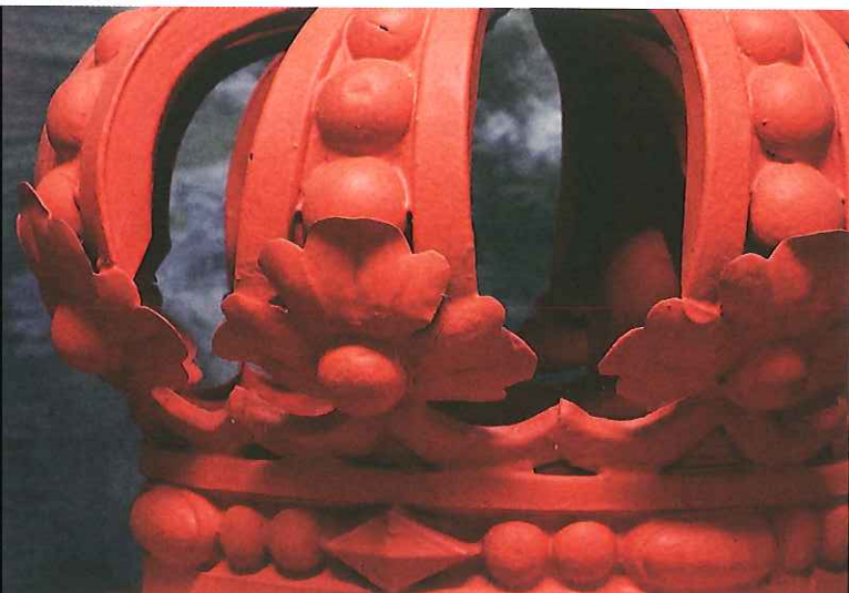
Red lead metal detail that will later be painted with linseed paint and gilded. No special permit is required when using red lead for professional purposes.
