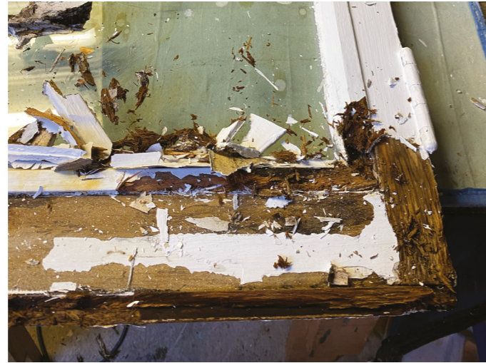
Window restoration uncovering rot - Joel Endersby Restoration.
