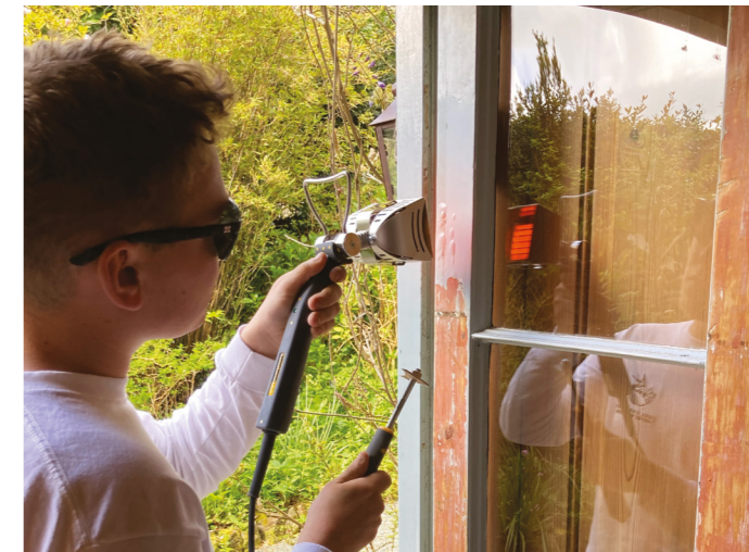
Paint stripping with infrared heat gun - Joel Endersby Restoration.
