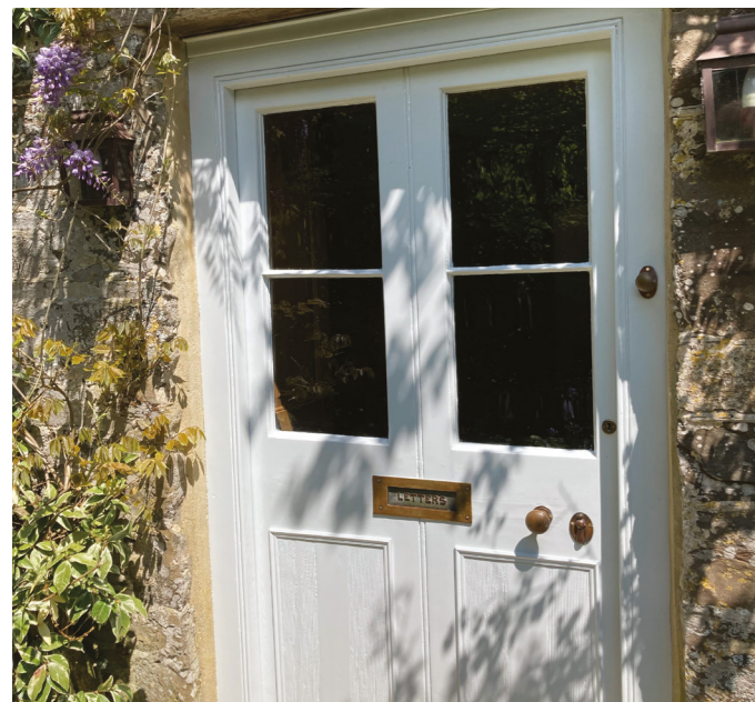
Door restoration completed with linseed oil paint - Joel Endersby Restoration
