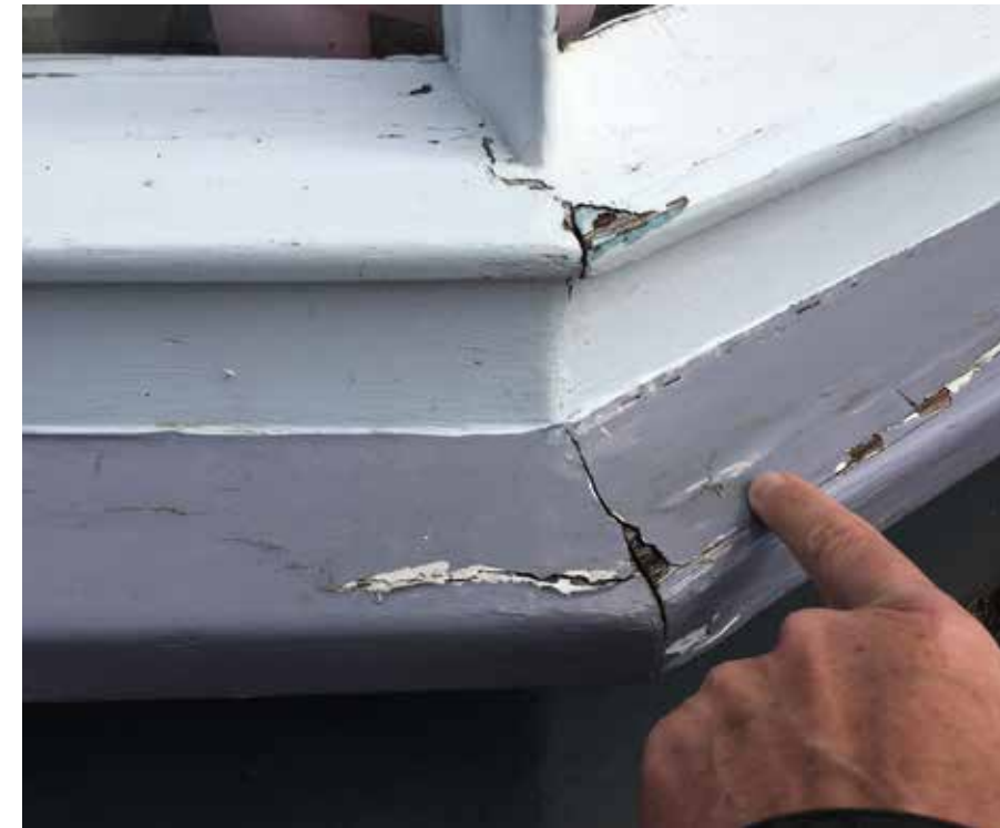
Bay window modern paint failure on Listed Building
