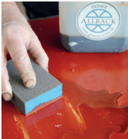
Wet-sanding with Primer will remove a wrinkled texture.
