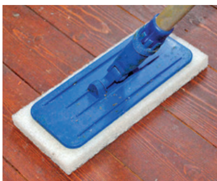
Linseed Oil Wax is easily applied with a scouring sponge such as the Scotch Brite brand.
