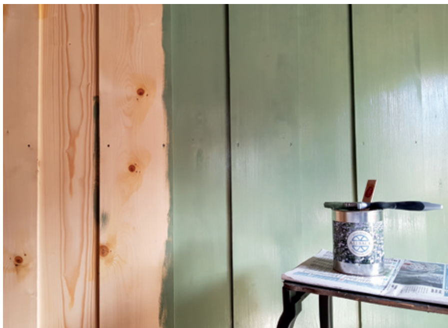
Seal knots with shellac as required to prevent staining. Paint outside and inside 2 - 3 coats. Colour: Wild Sage.
