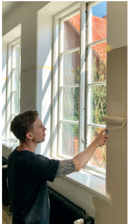
Fill and paint with Linus Wall Paint. Use a yarn roller or brush. Use a wide spackle knife or roller with Linus filler for skim coating (see page 19).
