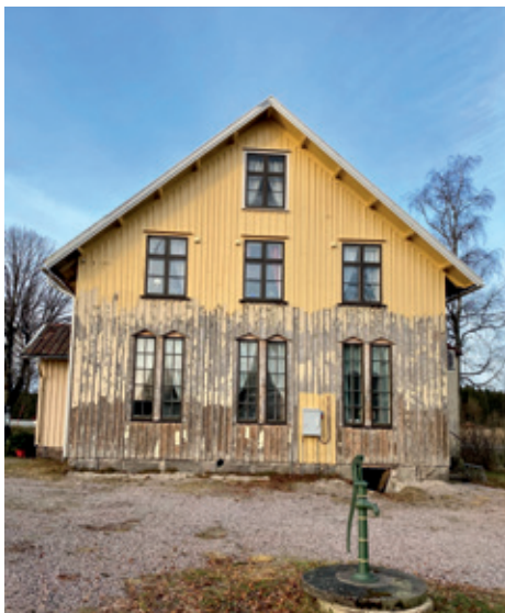
Nothing is too difficult for Allbäck Linseed Oil Paint. Scrape to a solid surface, clean, stain and finish painting.
