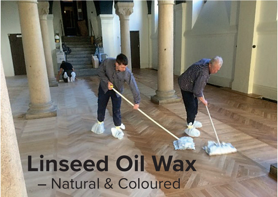
Pelarsalen, a hall at Lund University. Linseed Oil Wax on a new oak floor.
