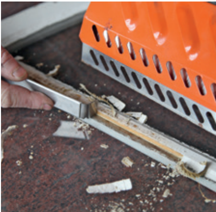
Putty Lamp to remove putty. It can also be used to remove paint to some extent.
