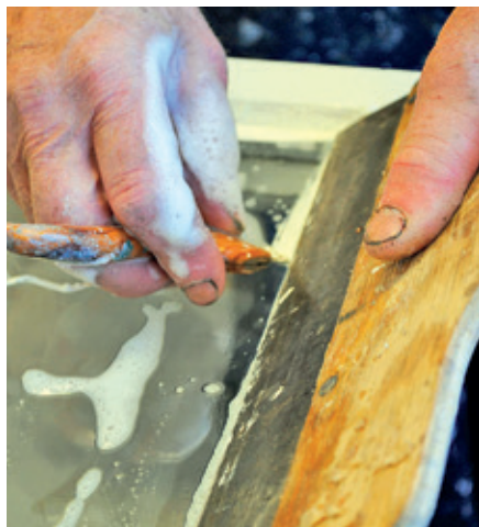
Cut the edges of the painted putty in a weak soap and water solution.
